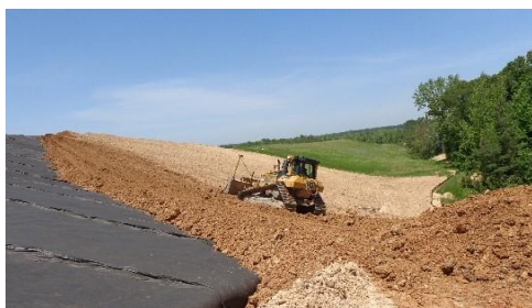
Geosynthetic Liner System Install
