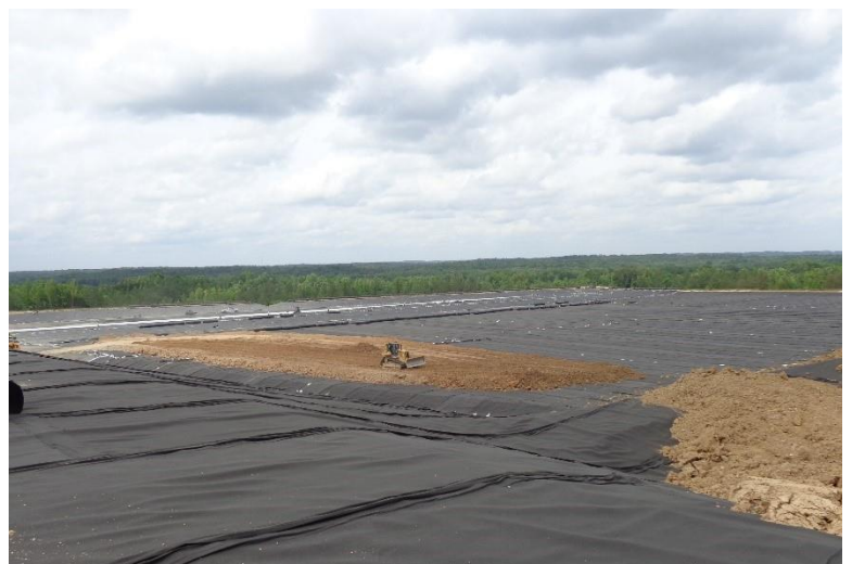
Cover Soil Placement
