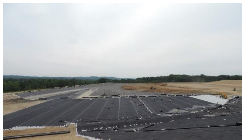
Liner Installation and Cover Soil
