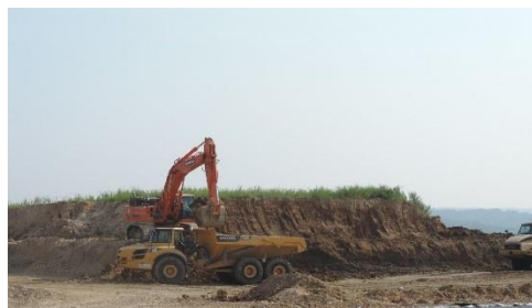
Cover Soil Excavation
