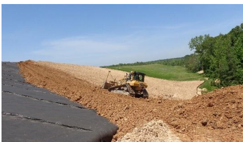
Geosynthetic Liner System Install
