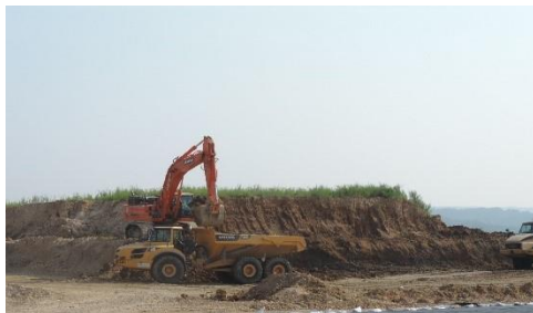
Cover Soil Excavation
