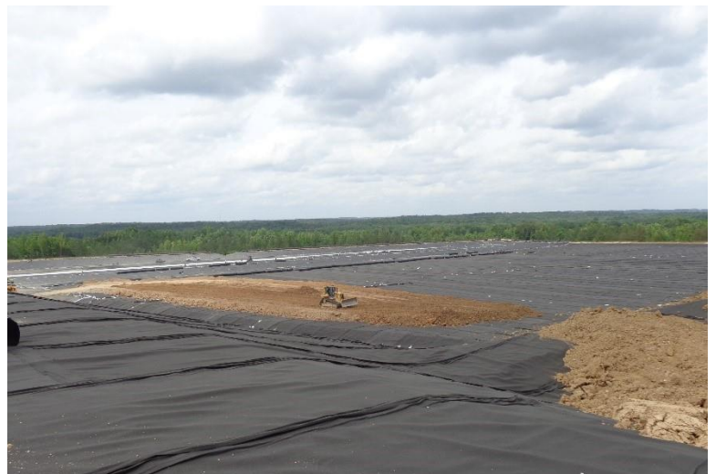
Cover Soil Placement
