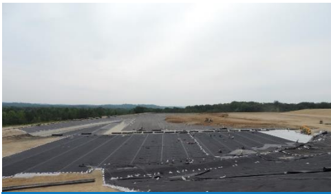
Liner Installation and Cover Soil
