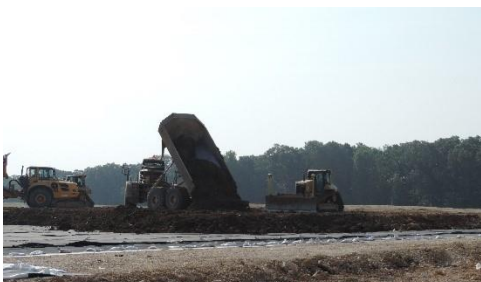
Liner Installation
