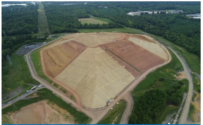
Final Grading & Seeding
