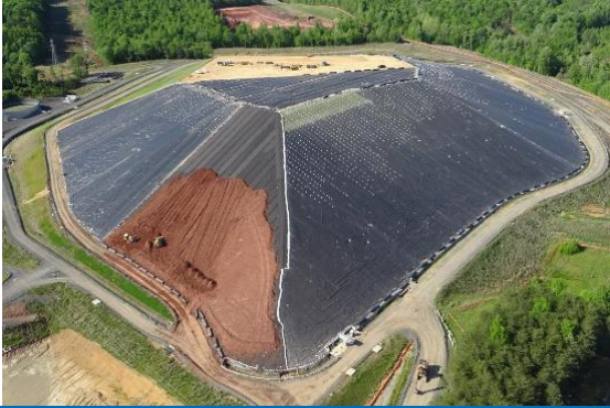
Liner Installation
