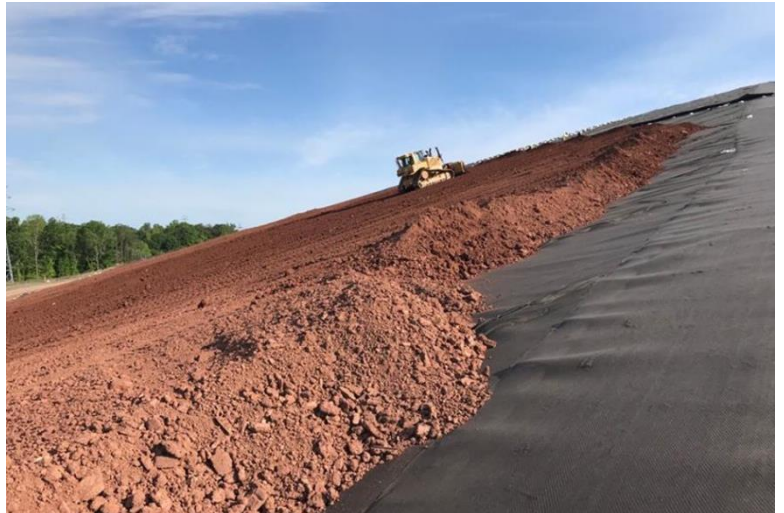
Cover Soil Placement
