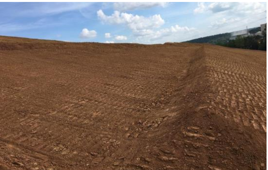
Tack-on Bench Construction
