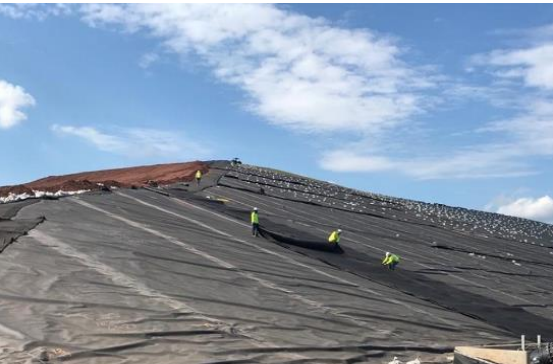
Geosynthetic Liner System Install
