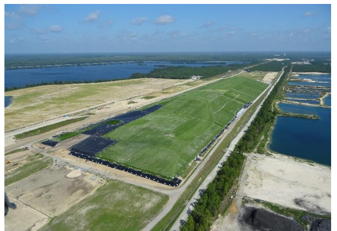
Final Stages of Completion
