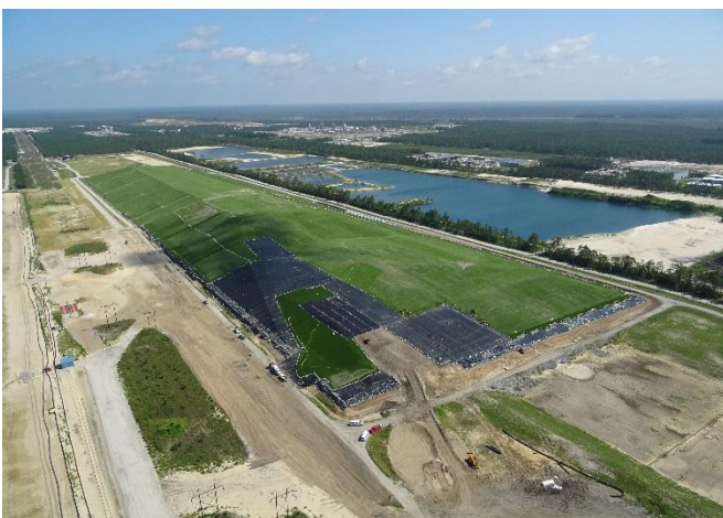
Liner/Closure Turf Installation
