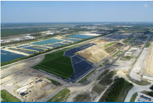
Initial line/Turf Installation
