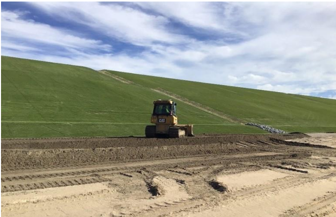
Grading of Landfill Cover
