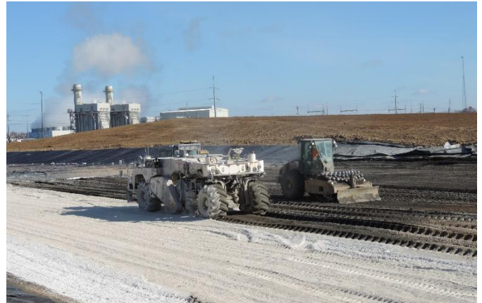
Basin Bottom Stabilization
