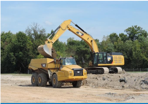
Excavating and Loading Cover Soil
