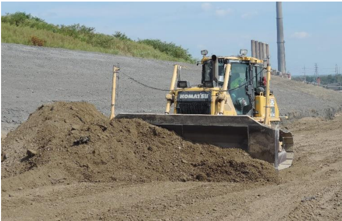
Placing Landfill Cover
