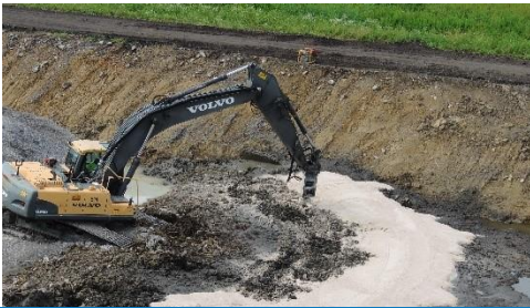
Lime Mixing Process
