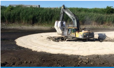
Lime Spreading
