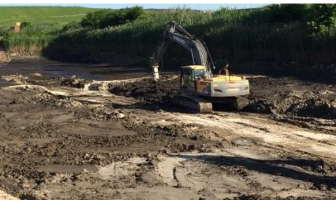
Ash/Soil Stabilization Progression
