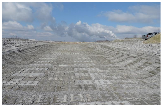
Completed Emergency Spillway #2
