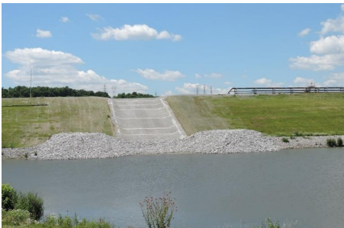
Completed Emergency Spillway #1
