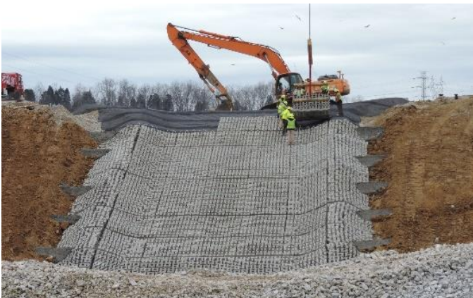
Articulated Concrete Block Installation
