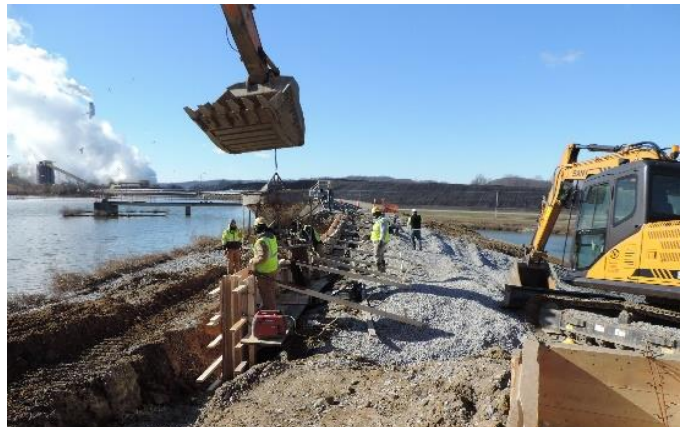
Cutoff Wall Installation
