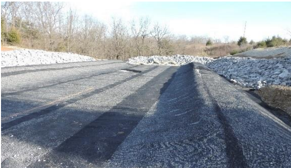
Aggregate and Geogrid Installation
