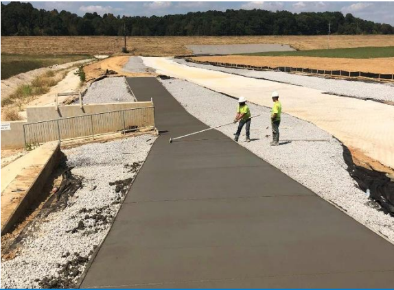
Spillway Concrete Installation
