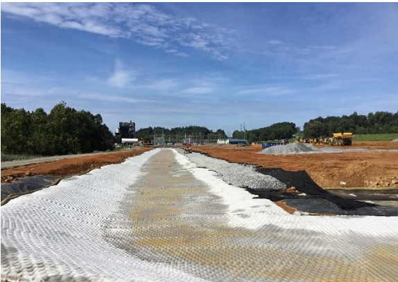
Fabric-Form Ditch Installation
