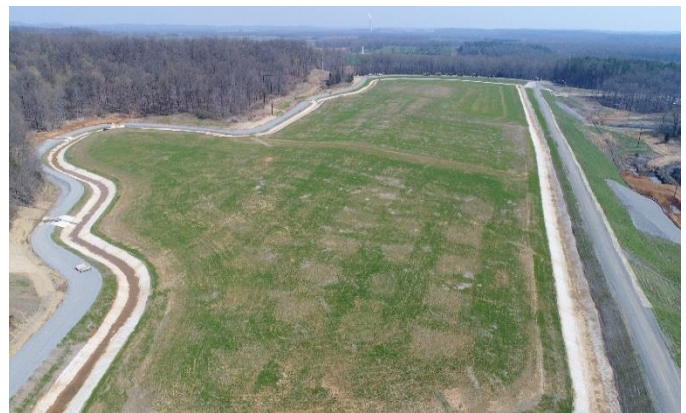
Final Basin Conditions
