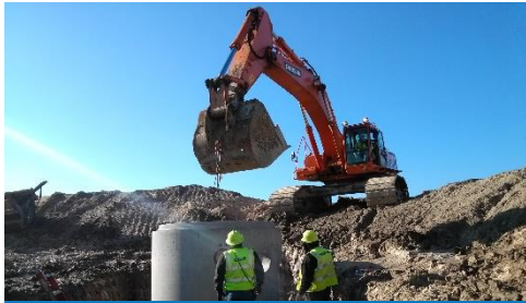
Manhole Installation
