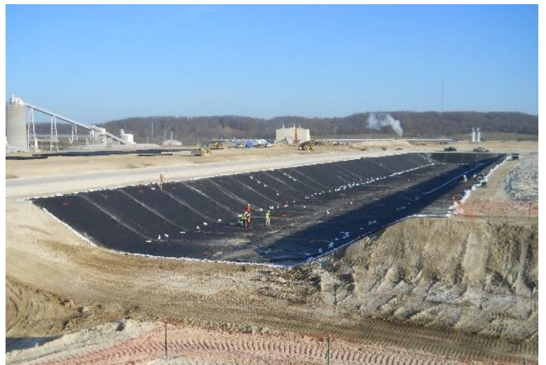
Liner Installation
