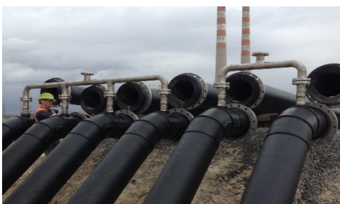
HDPE Pipe Installation
