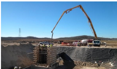
Cast-in-Place Concrete Installation
